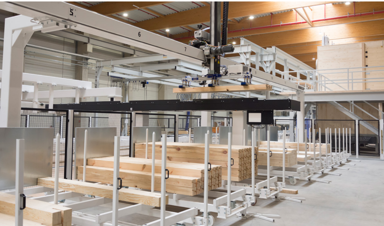
Pictures page 18: Gantry for feeding studs to the robot of the frame work station.
