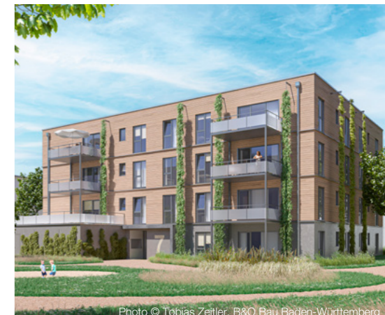
Picture above: Construction project by B&O Bau.
