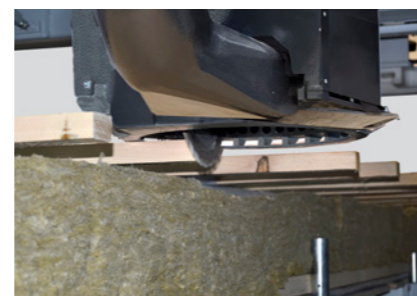
Formatting the roof battens
